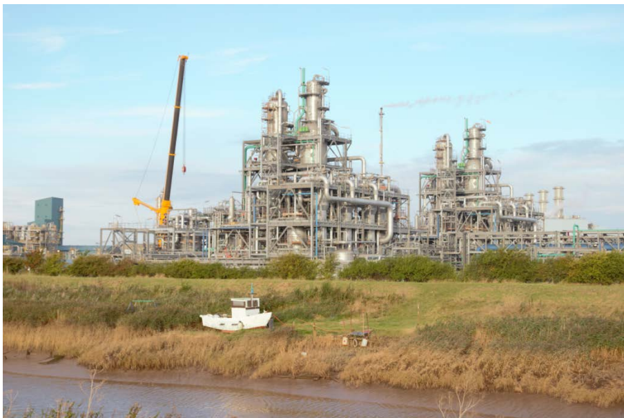
Mitsubishi site at Salt End
