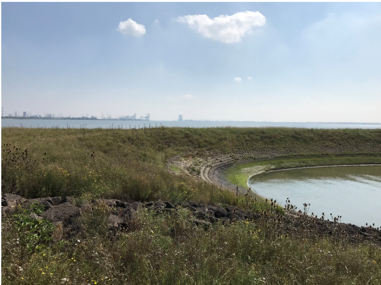
Bath berging spuisluis inside corner. Harbour of Antwerpen in the background
